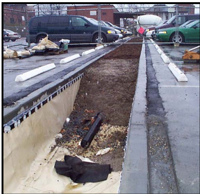
Figure C-4 Example of a parking lot retrofit where curbs were removed, allowing runoff to sheet flow into a bioretention area. This site is also a LUHPPL, so the bioretention area had to be lined.
