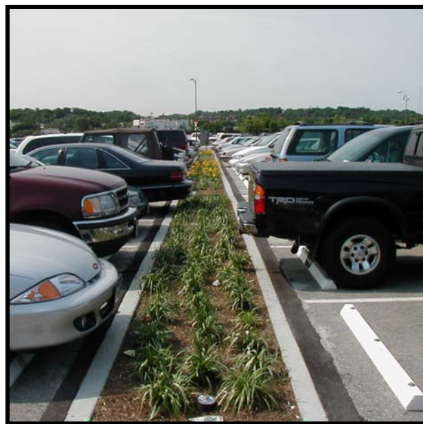
Figure C-4 Example of a parking lot retrofit where curbs were removed, allowing runoff to sheet flow into a bioretention area. This site is also a LUHPPL, so the bioretention area had to be lined.
